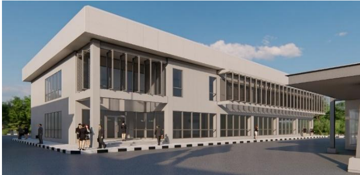
(a) DOH's Superintendent office at Ratchaburi toll Collection Point
