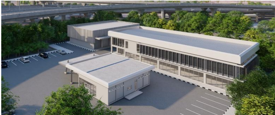
Operation And Maintenance Center
